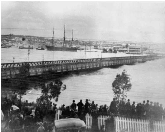
Figure 1. Brisbane, Australia – February 1893 – the Victoria Bridge before being heavily damaged by the floodwaters and floating debris. Note the local mounds upstream of the piers
