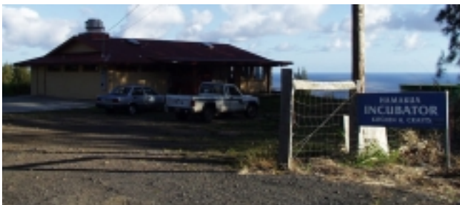
One of Hawaii’s shared-use kitchens.
