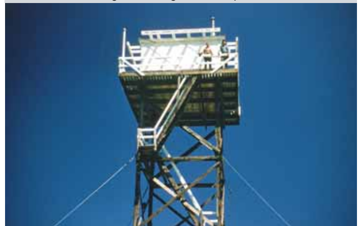
Bear Mountain Lookout. Example of tower lookout.
